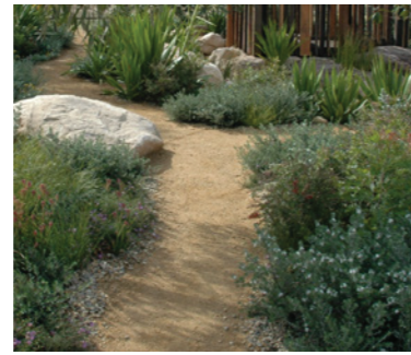
Stabilised Decomposed Granite
