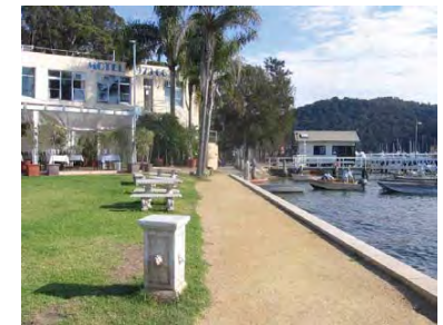
Public walkway to Pasadena waterfront
