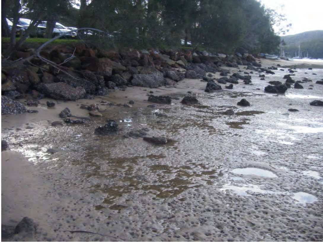
Fig 10 General view of foreshore erosion (looking west) showing mobilised rubble spread over inshore sand flat.
