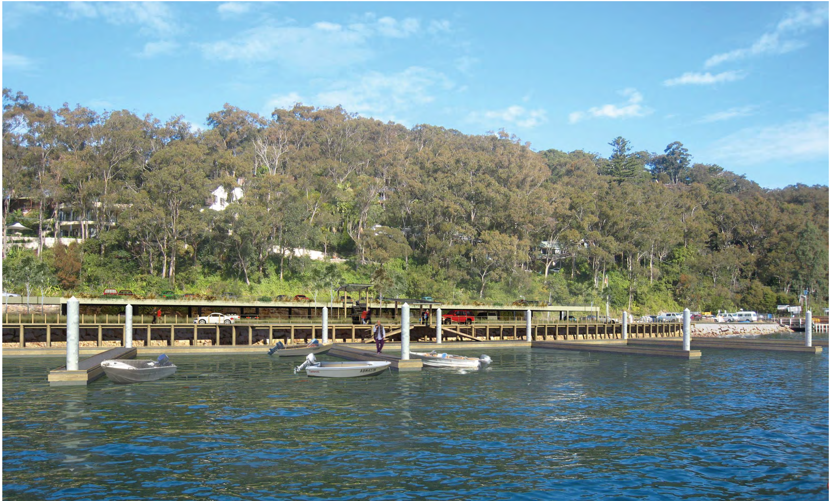
VIEW 2: Western car park on McCarrs Creek Road incorporating suspended deck - Artist Impression from Pittwater
