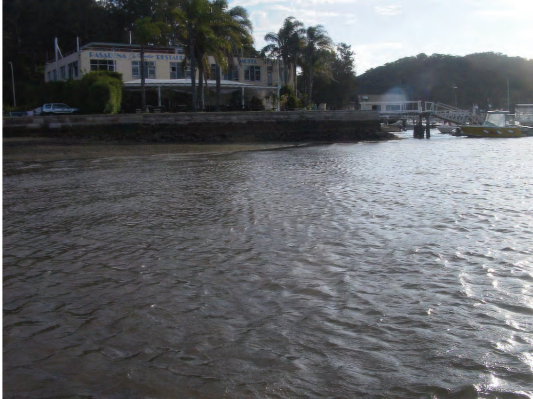
Fig 18 Eastern foreshore of Precinct 2 showing recently refurbished seawall.
