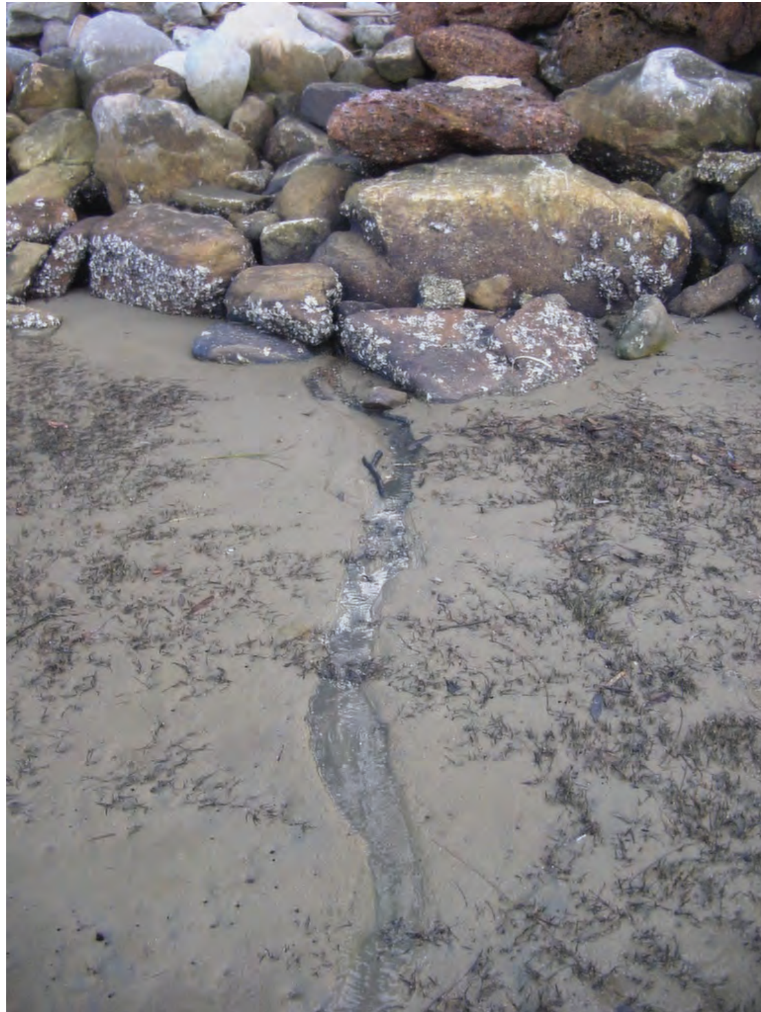
Fig 7 Car park seep drainage through the rock rubble
