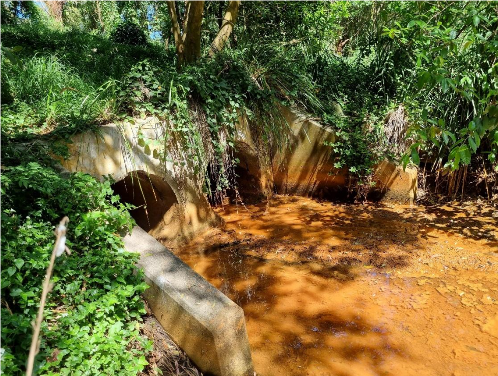
Photo 8 Culvert within the study area
