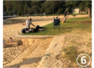
Formalised pedestrian access and retaining wall to beach
