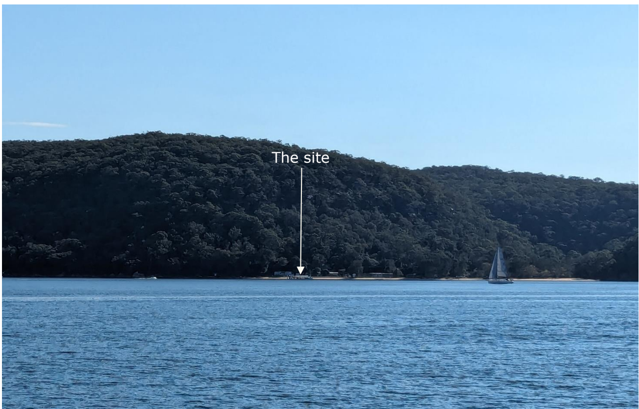
Figure 6-15 View from waterway to the site (Source: Worley Consulting, 2023)
