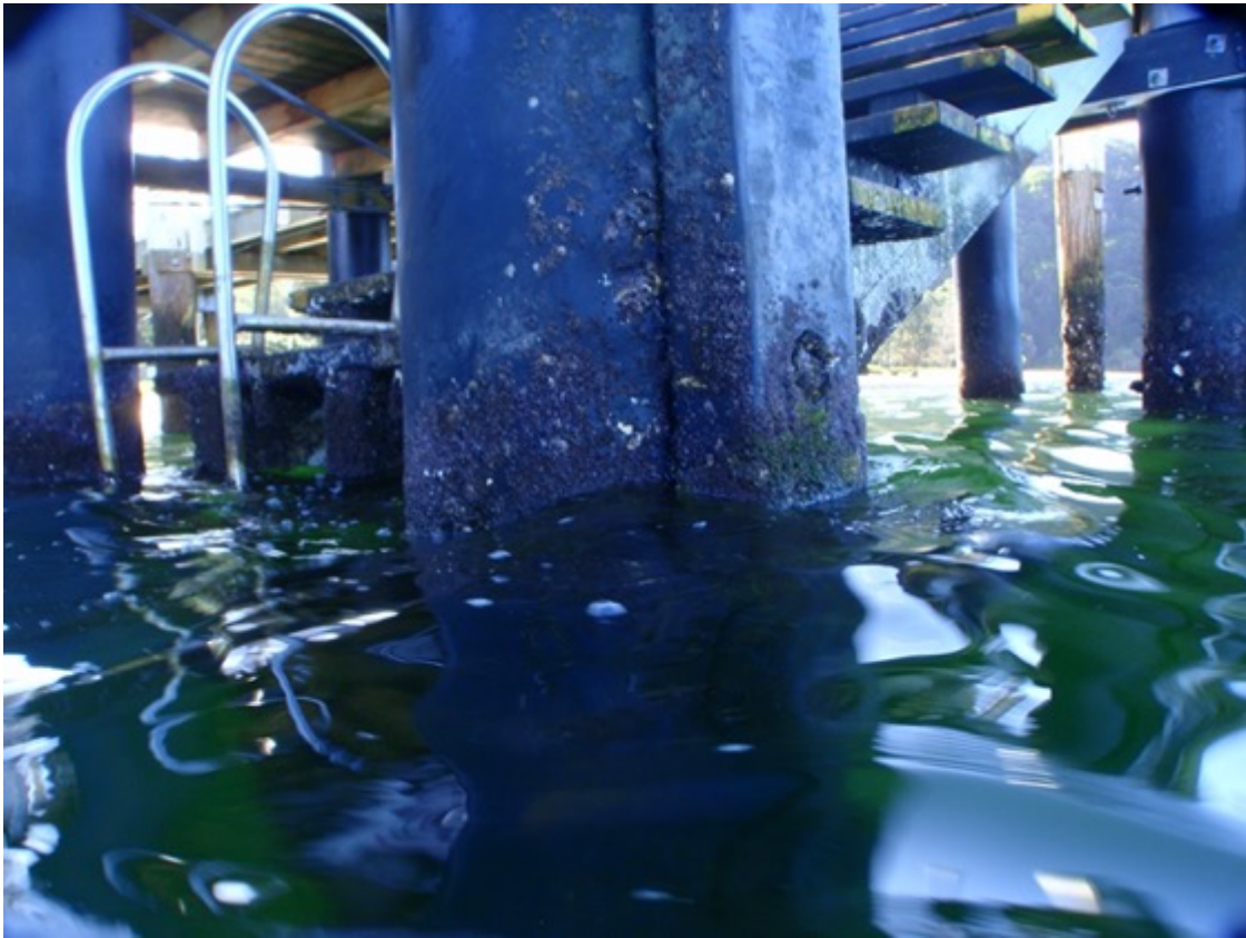
Figure 15 Little to no oyster growth on HDPE sleeved piles.
