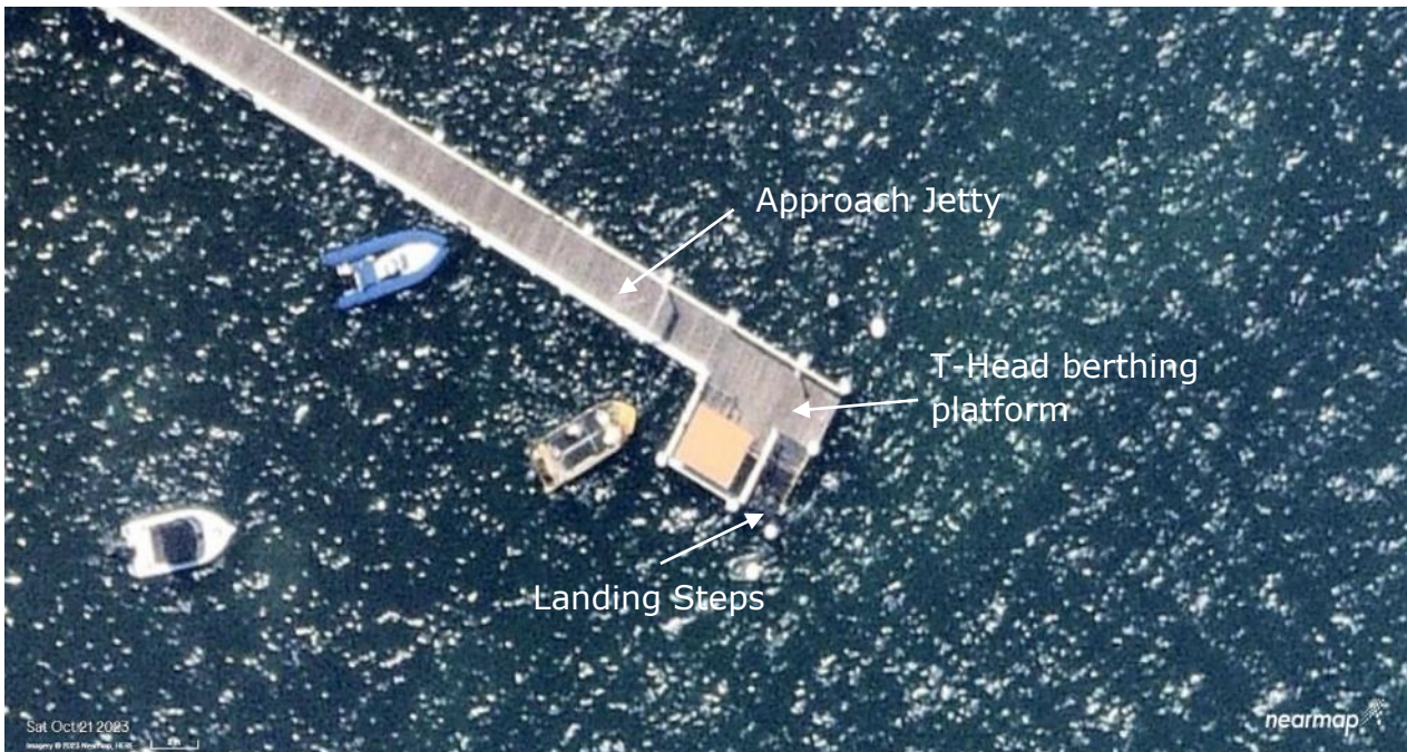
Figure 1-2 Currawong Wharf layout and features (Source: Nearmap, 2024)
