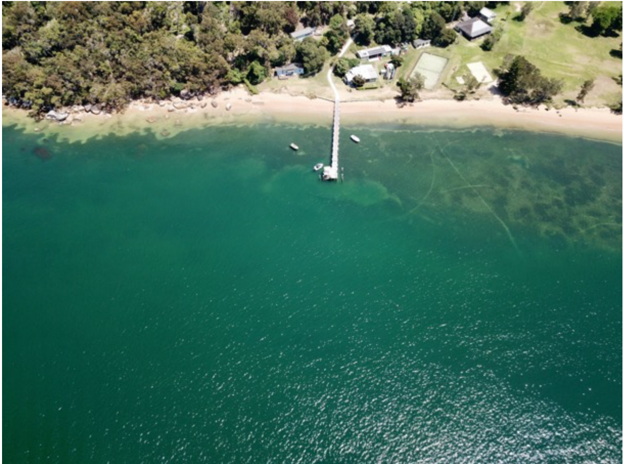
Figure 1 High tide aerial view of Currawong Beach and Public Wharf Facilities 1 February 2022.
