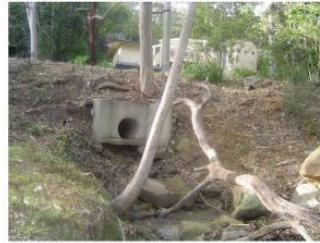
Photo 3. Stormwater outlet in Algona Reserve
