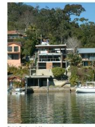
Photo 1: Development of foreshore area.
